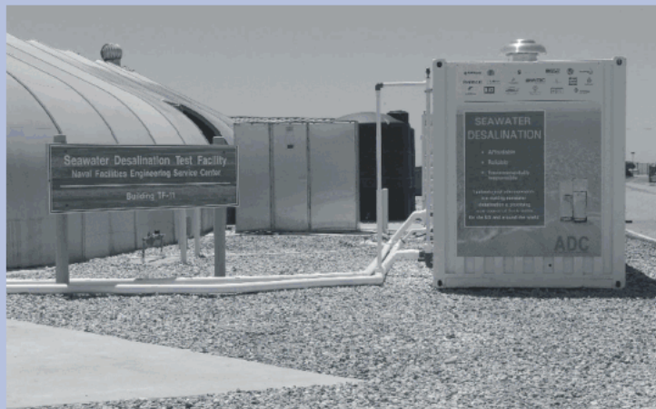
The ADC containerised demonstration system at the US Navy's Seawater Desalination Test Facility in Port Hueneme, California.
